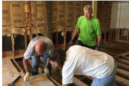
UM Men install new floor boards on a flooded home.
