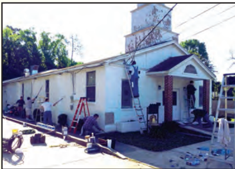
Tool Belt members repaint the exterior of Mount Moriah UMC.
