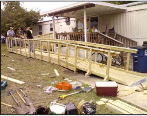
Men of Wylie (Texas) UMC build a handicap ramp.
