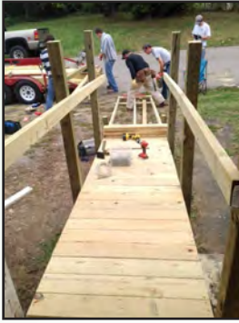
Scouts build a handicap ramp for Dianne Young.
