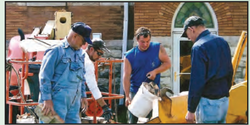
Men remove and replace the chimney of Earlville UMC.
