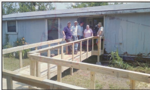
Wylie men complete a handicap ramp.
