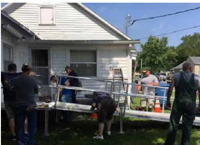
Members of Christ's Community UMC build ramps for people with handicapping.
